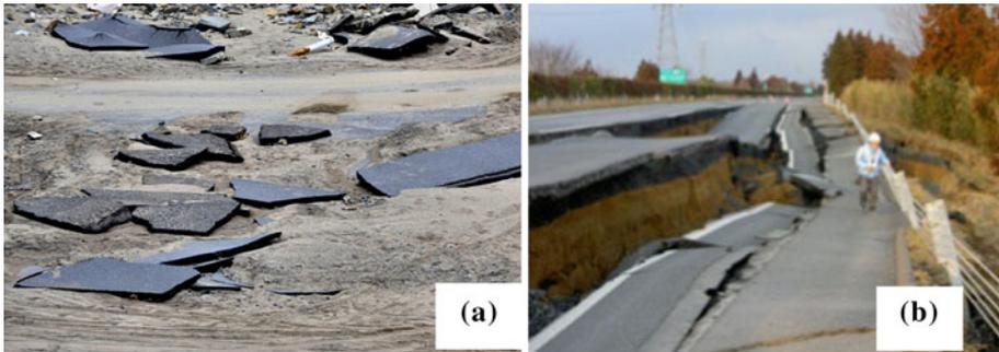
**Fig. 17** Damaged roads due to 2011 Tōhoku earthquake, Japan (Photo: **a** <http://www.tokyophotographers.com/2011/03/37-frames-great-tohoku-earthquake-tsunami-2011-japan-the-black-mouth-1.html> and **b** <http://buyjapanese.jp/about-japan/do-you-want-to-know-how-fast-japan-is-recovering-from-the-earthquake/>)
