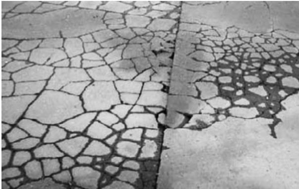
**Fig. 32** Minor cracks on road surface due to Tokachi-Oki earthquake (Tung 2004)
