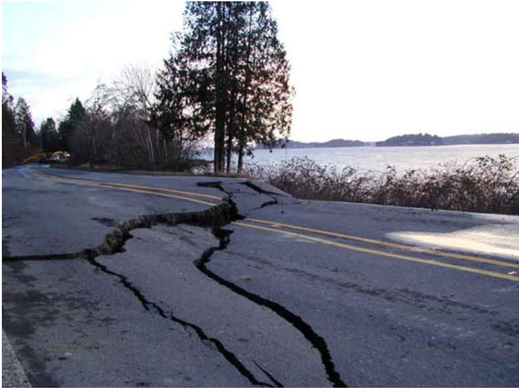
**Fig. 27** Road damage at Sunset Lake, Tumwater, from the 2001 Nisqually earthquake (Photo: [http://en.wikipedia.org/wiki/2001\\_Nisqually\\_earthquake](http://en.wikipedia.org/wiki/2001_Nisqually_earthquake))
