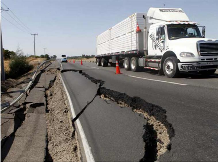
**Fig. 25** Road damage due to Chile earthquake 2010 (Photo: [http://www.channelnewsasia.com/photosgallery/gallery\\_20100228095431.htm](http://www.channelnewsasia.com/photosgallery/gallery_20100228095431.htm))
