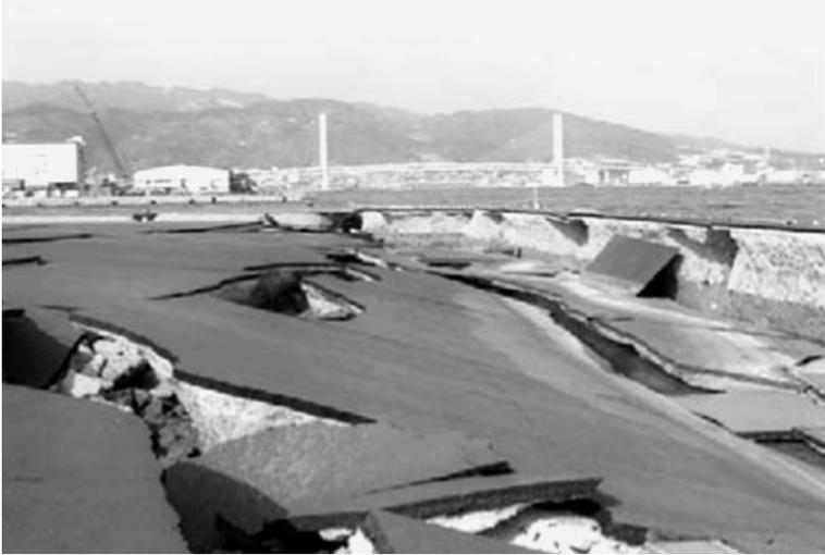
**Fig. 1** Road structure collapse due to Kobe earthquake (Tung 2004)
