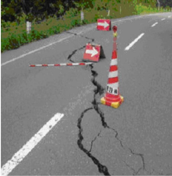
**Fig. 29** Cracks of Route 397 in Ohfunato due to Miyagi-Oki earthquake (DCRC 2003)
