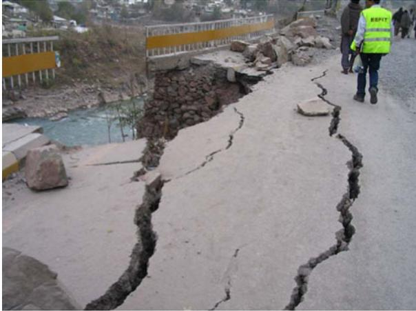
**Fig. 10** Damage of road due to Muzaffarabad earthquake (Navin and Matthew 2006)
