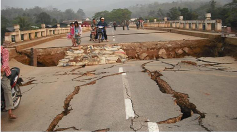
**Fig. 7** Damage of bridge approach road due to Myanmar (Burma) earthquake 2001 (CBC 2011)
