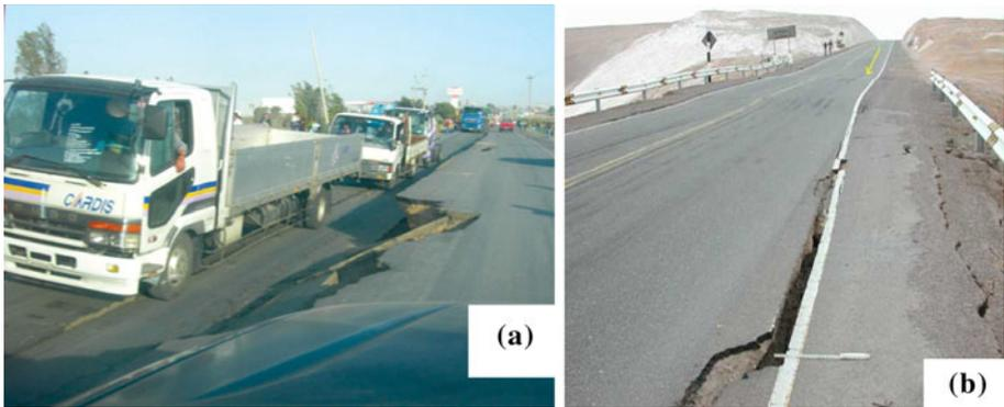
**Fig. 18** Damaged roads due to Peru earthquake 2007 (Photo: **a** Pan-American Highway (MCEER 2007) and **b** Highway damage (GEER 2008))
