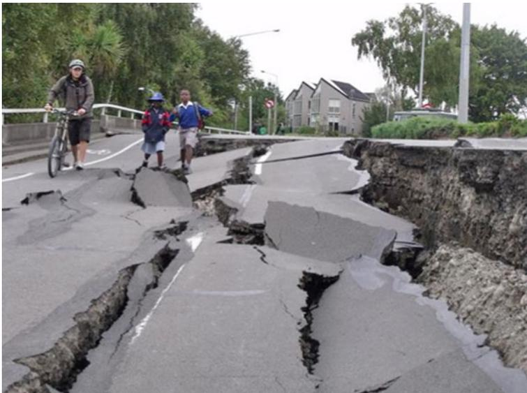
**Fig. 15** Damaged road due to Christchurch earthquake (Photo: <http://eqchch.wordpress.com/2011/02/25/canterbury-christchurch-earthquake-damage-2011/>)
