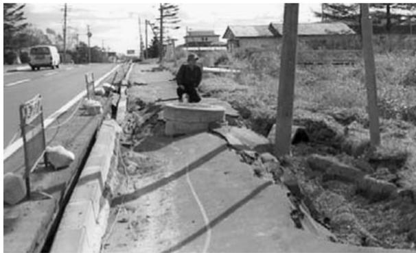
**Fig. 22** Severe defect on road surface due to Hokkaido Toho-Oki earthquake (Tung 2004)
