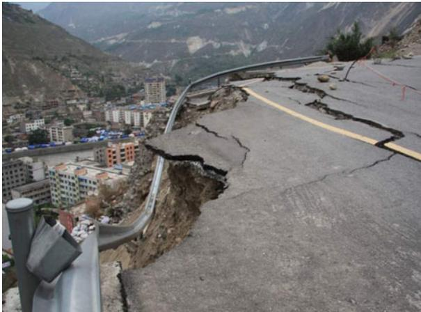
**Fig. 9** Road damage in Yingxiu due to Wenchuan earthquake (Zifa 2008)
