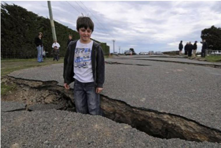
**Fig. 26** Damaged road due to Canterbury earthquake 2010 (Photo: <http://www.natural-calamity.info/earthquake-destroyed-about-500-buildings-in-chrishchurch/>)
