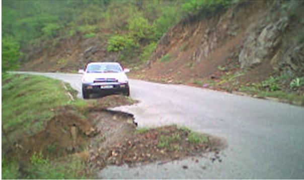
**Fig. 23** Bostan–Jasenovik road is damaged in some parts and ditches are covered with stones and earth (EDARP 2002)
