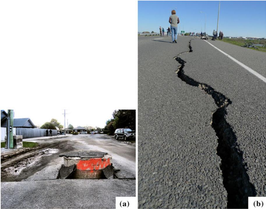
**Fig. 30** Low to moderate damaged roads due to 2010 Canterbury earthquake (Photo: [http://en.wikipedia.org/wiki/2010\\_Canterbury\\_earthquake](http://en.wikipedia.org/wiki/2010_Canterbury_earthquake))
