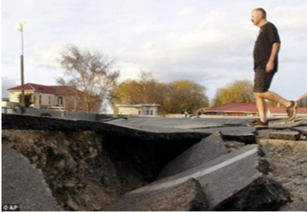
**Fig. 14** Damaged road due to Canterbury earthquake 2010 (Photo: <http://archive.wn.com/2011/03/07/1400/worldnaturaldisaster/>)
