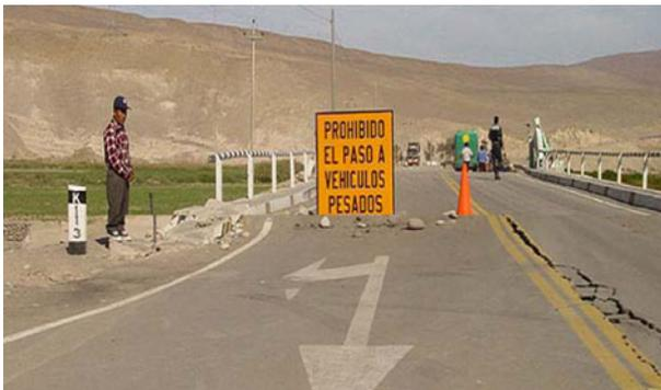
**Fig. 31** Settlement of bridge approach and cracking of road. Only one lane is open for traffic (Nakamura 2000)
