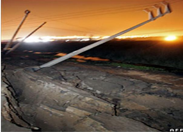
**Fig. 3** A damaged road in Southern Peru due to Peru earthquake (EERI Special Report 2007)
