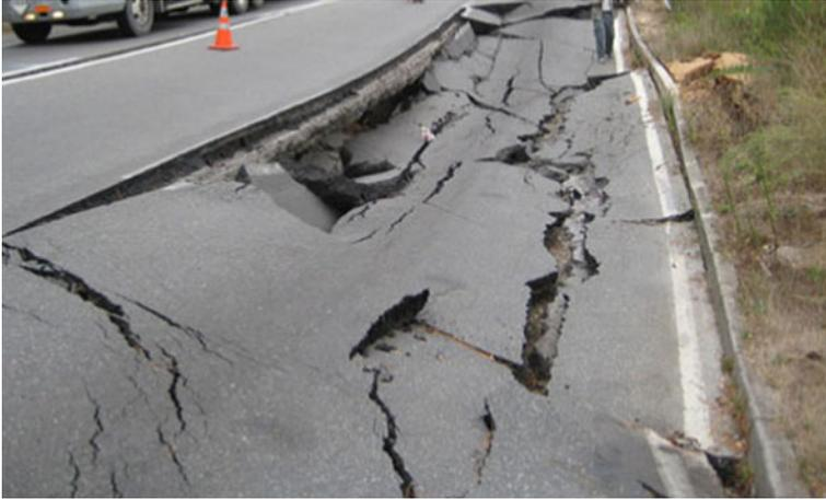
**Fig. 12** Damaged road due to Chile earthquake 2010 (Photo: <http://news.bbc.co.uk/2/hi/americas/8542112.stm>)
